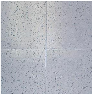
Newly installed VCT
